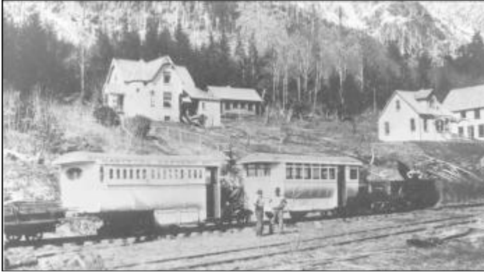
Hartford Eastern gas cars at Silverton. The car on the left is towing a utility trailer; the one on the right has a small snow plow attached to the front. Photo courtesy of Granite Falls Historical Museum.
